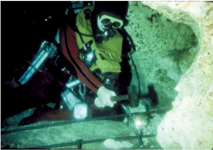
Jack Banbury driving rebar. Note the horseshoe collar, large heavy drop weights at his waist and plexiglas light head to the right. The large metal battery pack sits on the diver's hip.
