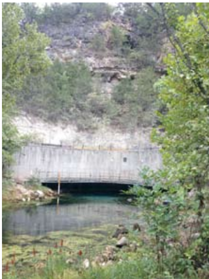
Roubidoux Spring - entrance at the base of the retaining wall. Photographer: Lori Bennett
