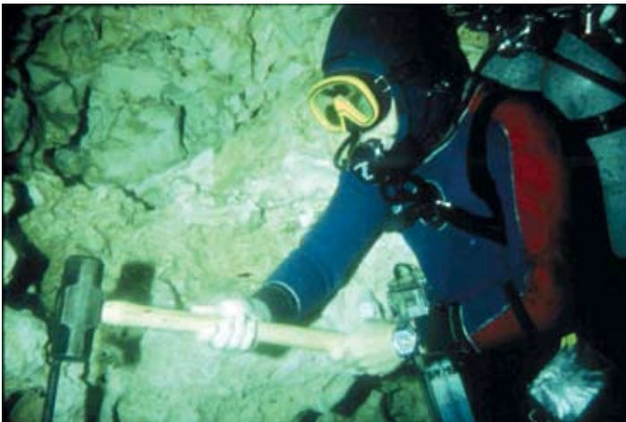
Tom Mount hammers rebar into place
