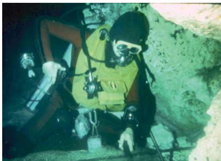
Jack Banbury setting rebar
