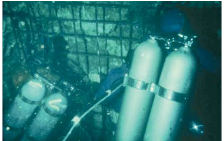
Divers setting the grate.
